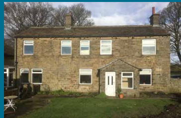
Existing farmhouse undergoing refurbishment 3 bedrooms 2 bathrooms
